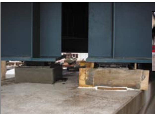
Chemnitz-Einsiedel viaduct, Blankenauer street: repairing bridge bearings
