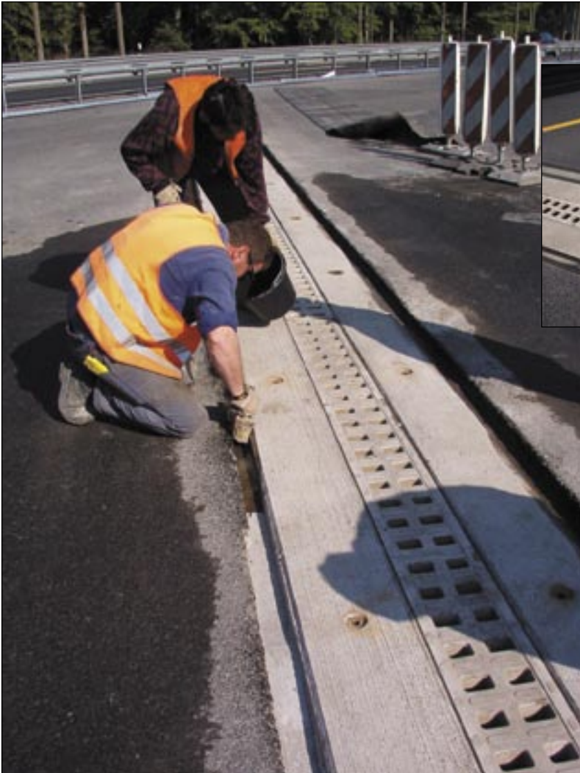
A2 Motorway, Hamm-Uentrop: Construction of transverse drainage channels
