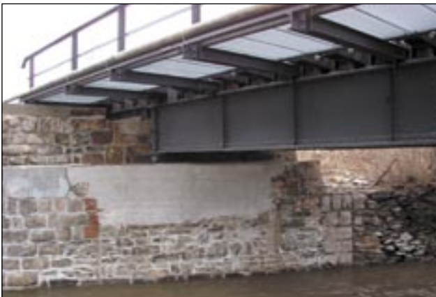
Chemnitz-Einsiedel viaduct, Blankenauer street: repairing bridge bearings
