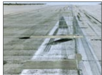
Leipzig/Halle Airport: Repairing concrete, runways and taxiways
