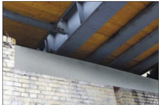
Metropolitan viaduct, Berlin, Sterndamm: repairing bridge bearings
