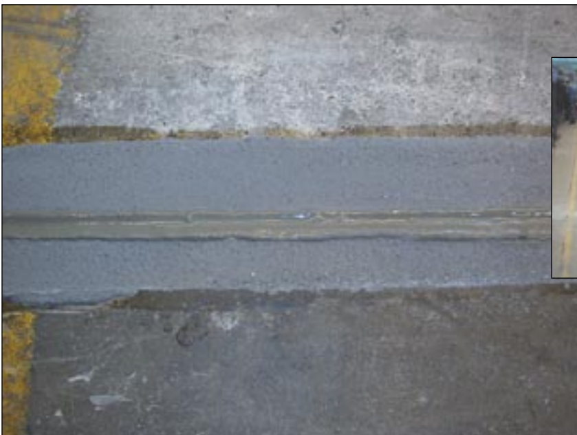
Left: Rheingas AG, Brühl: Repairing sliding gate
