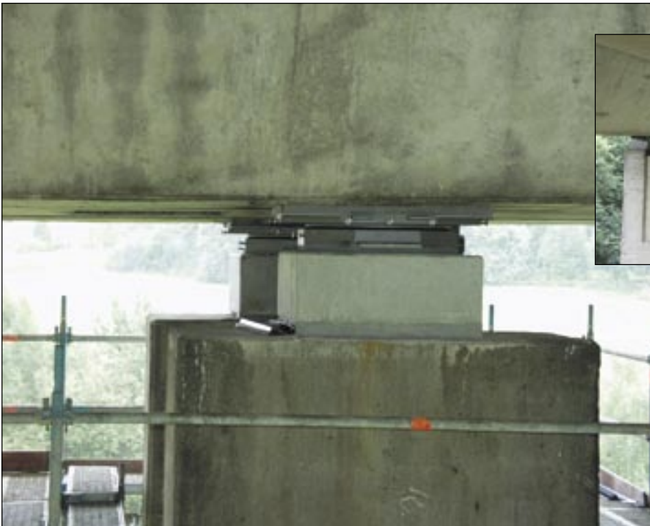
A7 motorway bridge, Uttrichshausen: Repairing bridge bearings
