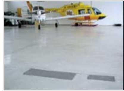
Mannheim Airport Repairing hangar floors
