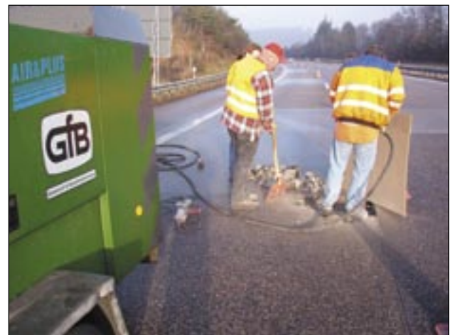
A3 Motorway, Neustadt/Wied: Improving the road surface
