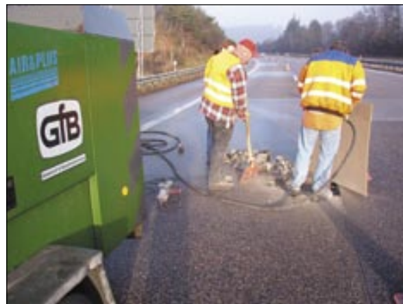
A3 Motorway, Neustadt/Wied: Improving the road surface
