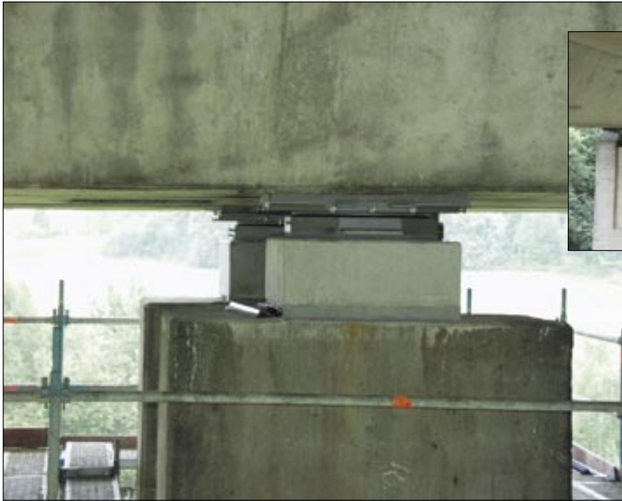
A7 motorway bridge, Uttrichshausen: Repairing bridge bearings
