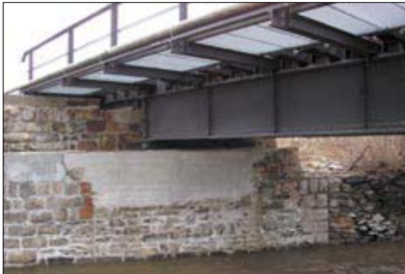
Chemnitz-Einsiedel viaduct, Blankenauer street: repairing bridge bearings
