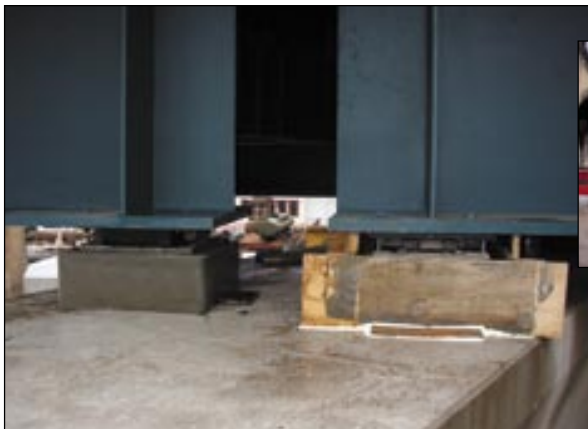
Chemnitz-Einsiedel viaduct, Blankenauer street: repairing bridge bearings
