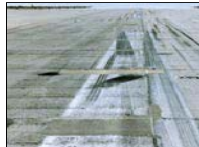
Leipzig/Halle Airport: Repairing concrete, runways and taxiways
