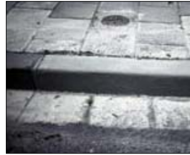
Repairing the kerbs with SILIKAL® Mortar R 17
