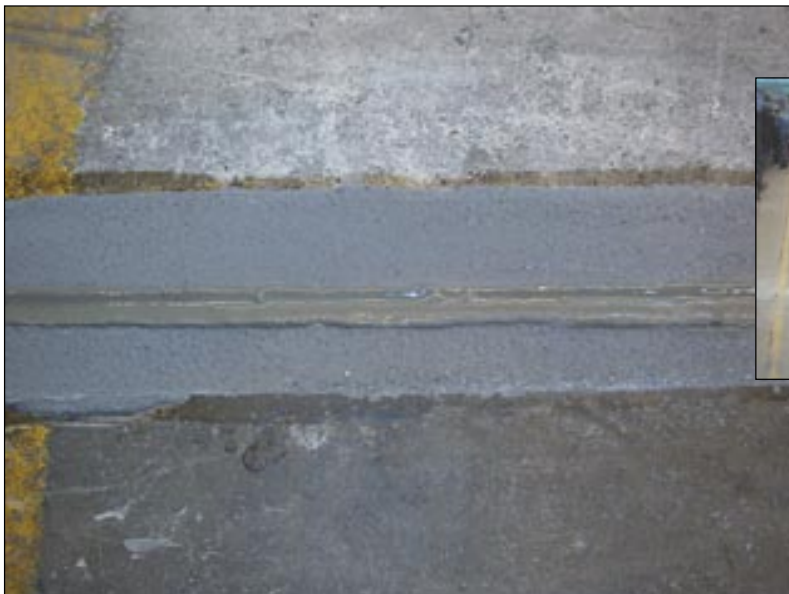
Left: Rheingas AG, Brühl: Repairing sliding gate
