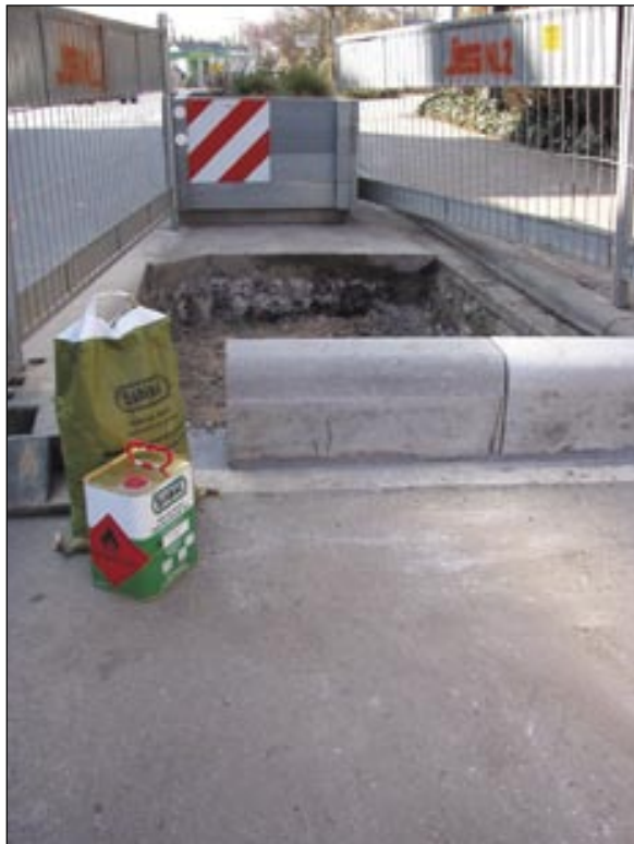
Ladenburg, Schriesheimer street: Building a flower bed with kerb bricks stuck to the asphalt with SILIKAL® Mortar R 17
