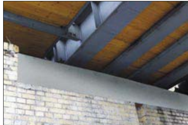
Metropolitan viaduct, Berlin, Sterndamm: repairing bridge bearings
