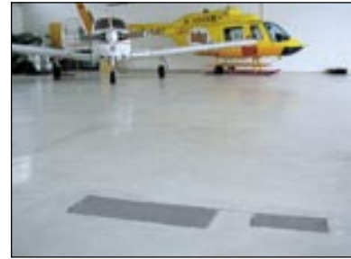
Mannheim Airport Repairing hangar floors
